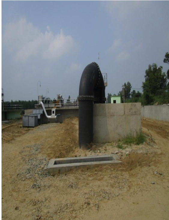
MAIN PUMPING STATION INLET:-
