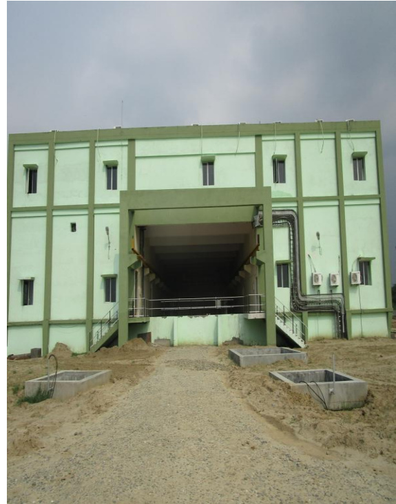
MAIN PUMPING STATION:-
